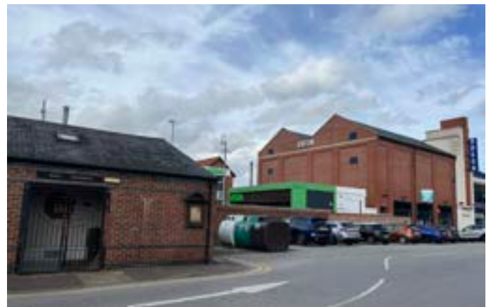
Areas with blank or lack of frontage, minimising overlooking and passive surveillance.
