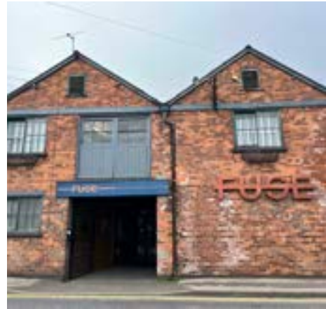
Converted warehouse building into a gym
