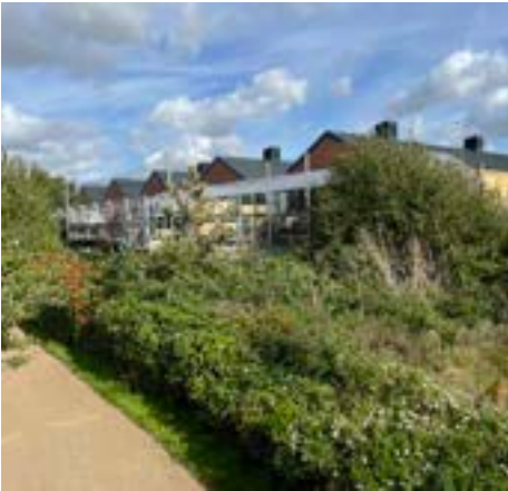
The rear of The Maltings Retail Park
