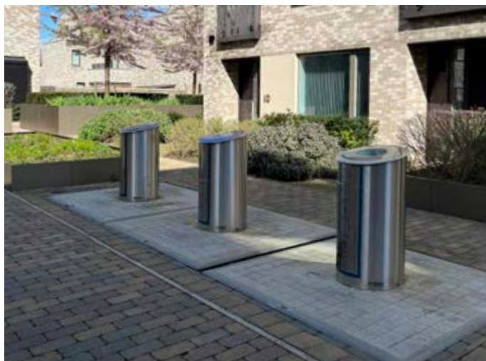
Underground bins in a new residential development with segregated collection of waste, recycling and compostable waste
