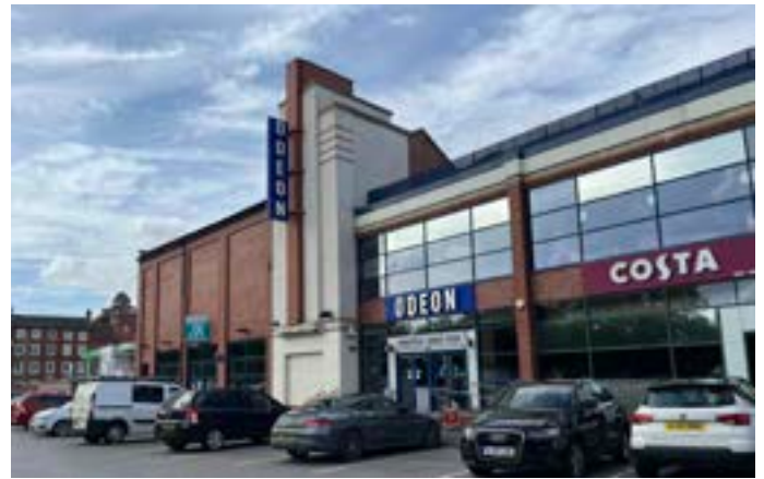
Lack of active frontage, with parking up to the building line of the Odeon and Costa in London Road Car Park.
