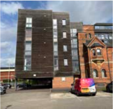
New build extension on Warwick and Richardson Brewery conversion
