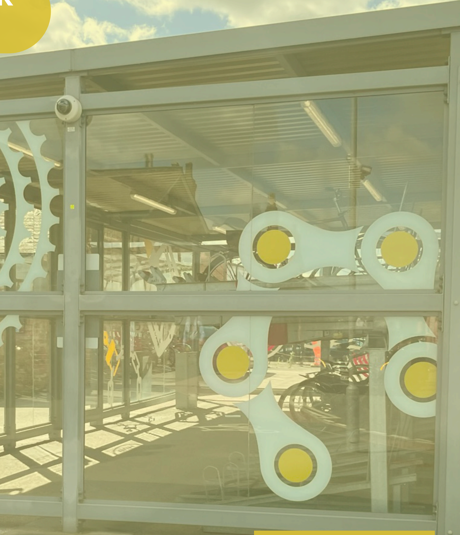
Cycle shed at Newark Northgate Station
